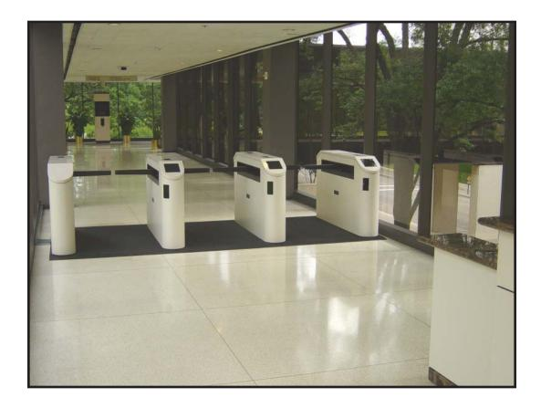
The Designed Security, Inc. **ES831 bi-directional optical turnstiles** with hands-free barrier arms enhance the security of access control systems. The ES831 provides a visual as well as a psychological barrier while communicating to pedestrians that authorization is required to gain access to a facility or area.
